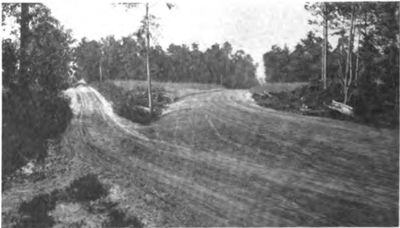
AN OLD ROAD AND THE NEW
