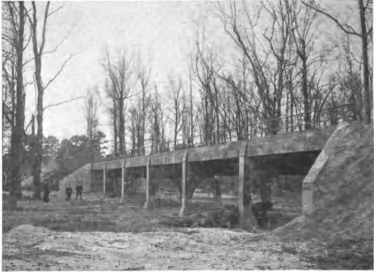
EDGECOMBE HAS MORE THAN FORTY CONCRETE BRIDGES
