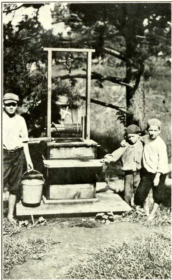
No. 25.—Well supplying water to one of the mills, Haw River, N. C. Notice the privy just above the well, x
