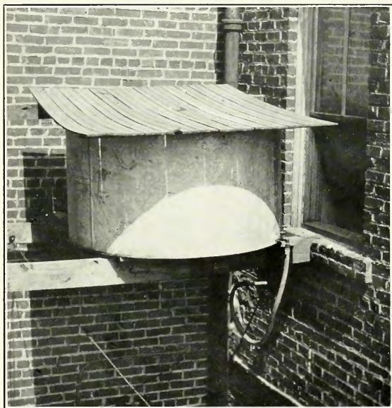
No. 3.—Tank of Burlington Bottling Works. Overflows daily.
