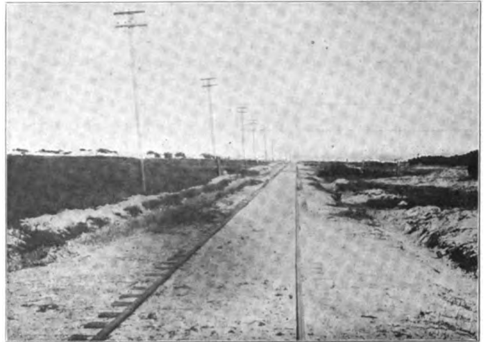
TRACK LAID IN SAND—SULLIVAN'S ISLAND.
