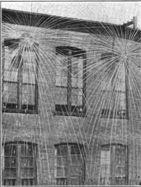
SPRAY FOR COOLING MILL.
