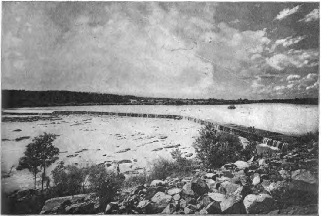
DAM ACROSS BROAD RIVER FOR COLUMBIA CANAL.
