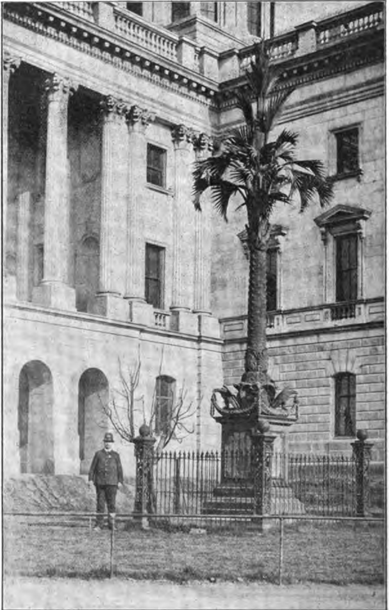
MONOLITH COLUMNS—22 TONS EACH. SOUTH CAROLINA GRANITE.
