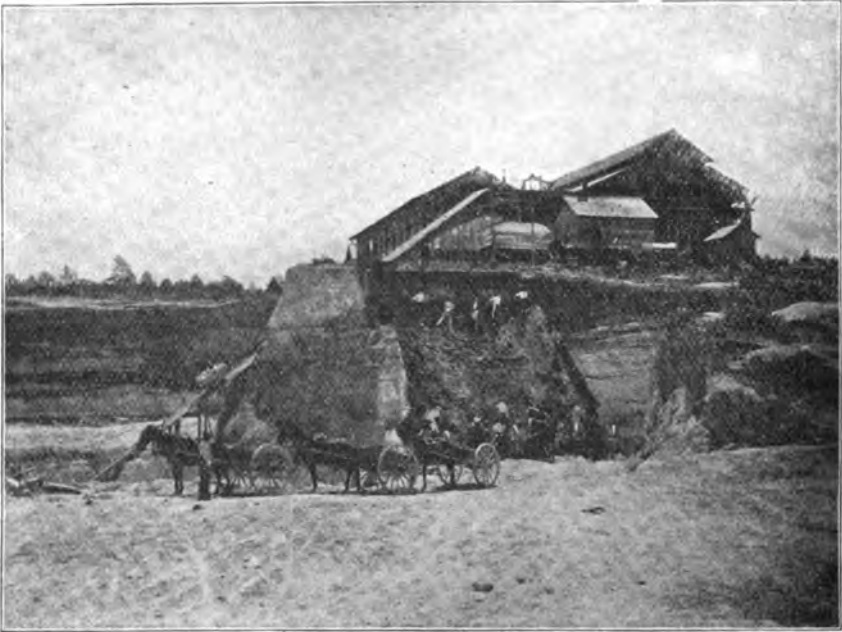
SEDIMENTARY KAOLIN MINE—REMOVING THE OVERBURDEN.
