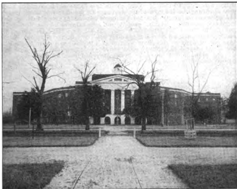
MILLS BUILDING, STATE HOSPITAL FOR THE INSANE—FOUNDATIONS LAID IN 1822.
