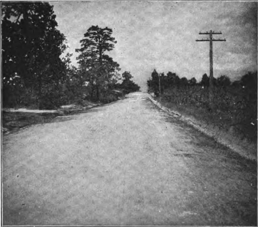
A COMPLETED SAND-CLAY ROAD.
