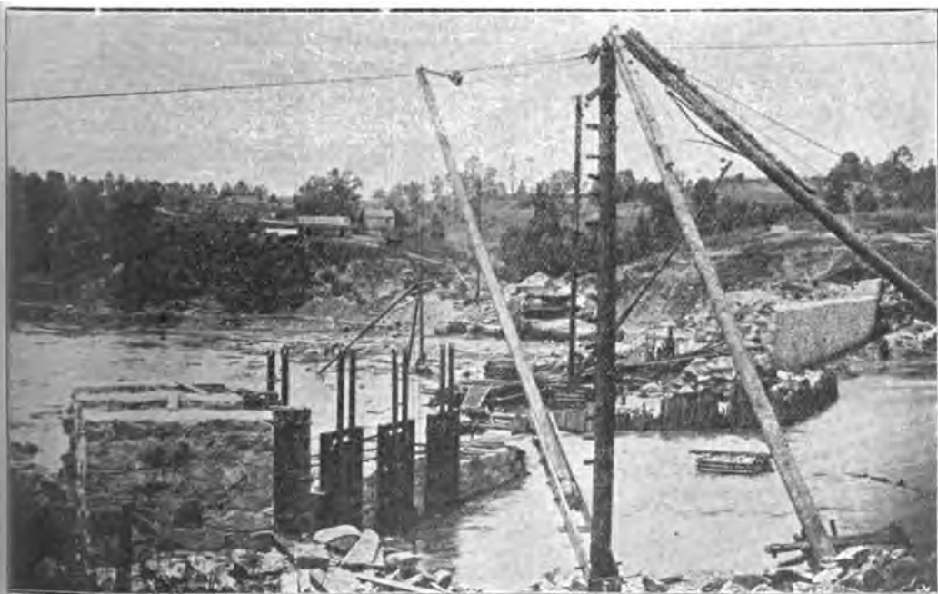
CONSTRUCTING A POWER DAM.
