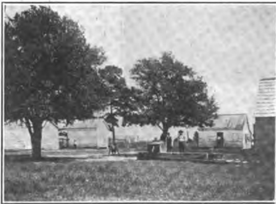
ARTESIAN WELL IN BARNYARD ON CREIGHTON PLANTATION.
