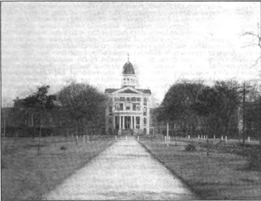
MAIN BUILDING, STATE HOSPITAL FOR THE INSANE—COMPLETED IN 1885.
